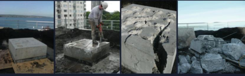
Rock Breaking - No blasting, No noise, No vibration, Easy Removal Breaking boulders, both big and small, in densly populated residential areas
